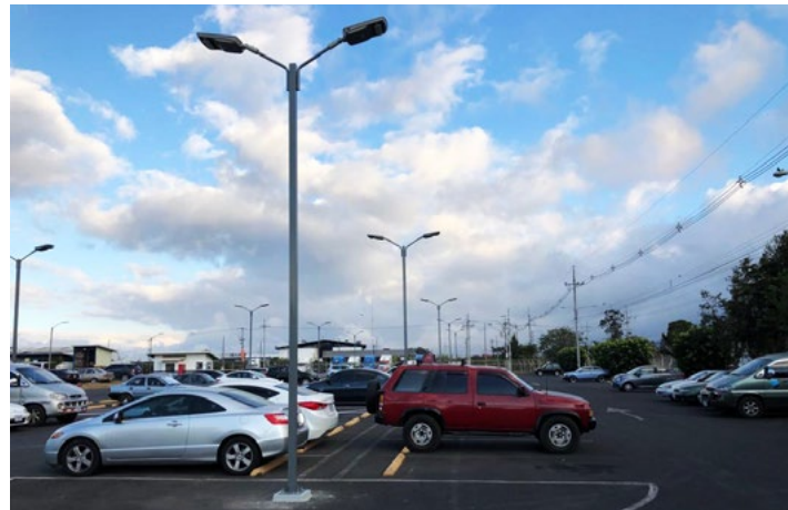
Kimberly. Clark Company Costa Rica Parking Lots Lighting Project
