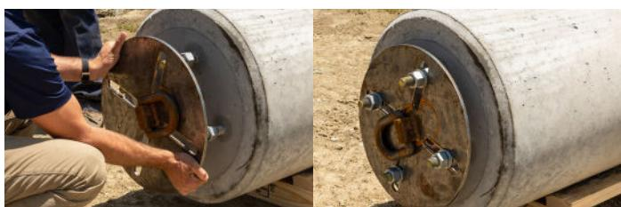
**1** Attach lifting bracket to pole base.
